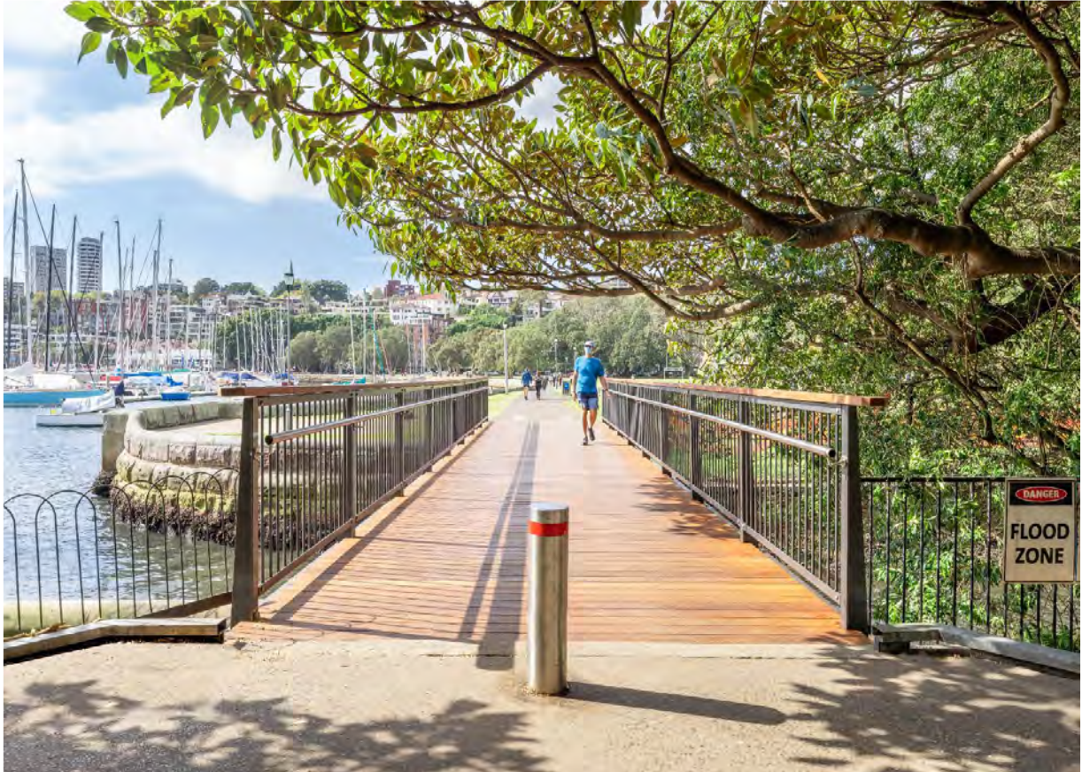
Image: Rushcutters Bay Park Bridge, City of Sydney
