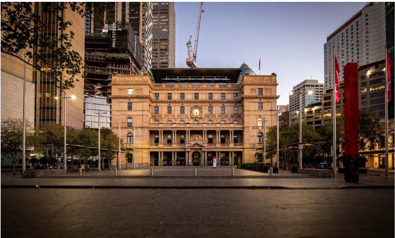
Figure 5. Customs House, Circular Quay – Photo by Katherine Griffiths / City of Sydney
